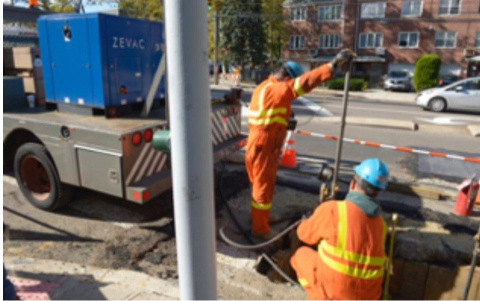
Figure 8: Crews working with ZEVAC
